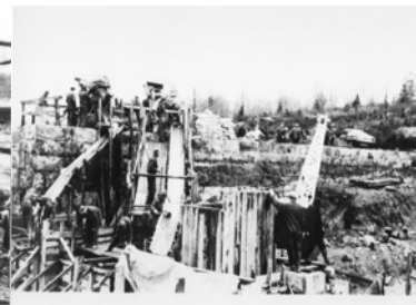
Pouring the sluice tunnel - 1939
