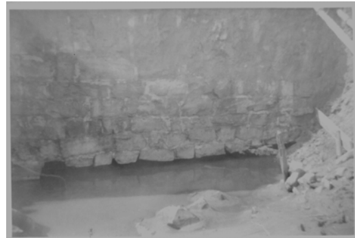
Water under the masonry core.
